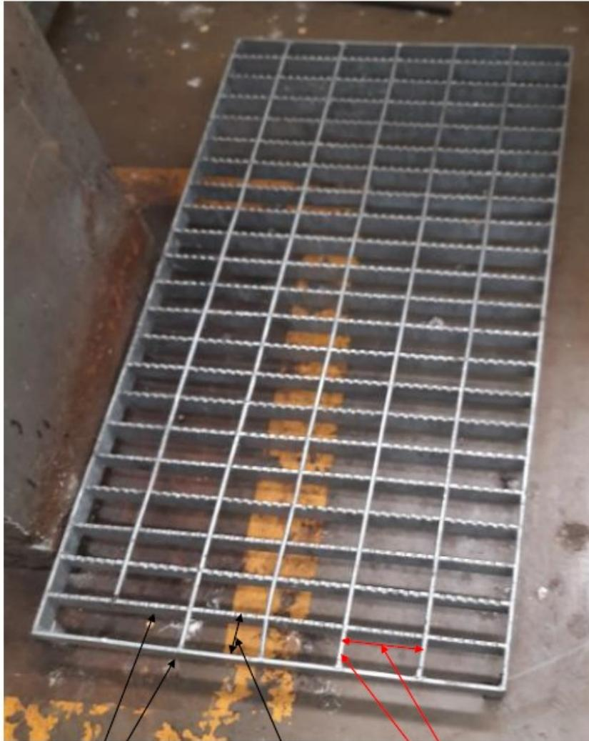
Horizontal and peripheral members shall be of 40mm x 5mm GI flat, spacing between the horizontal members shall be 50mm
